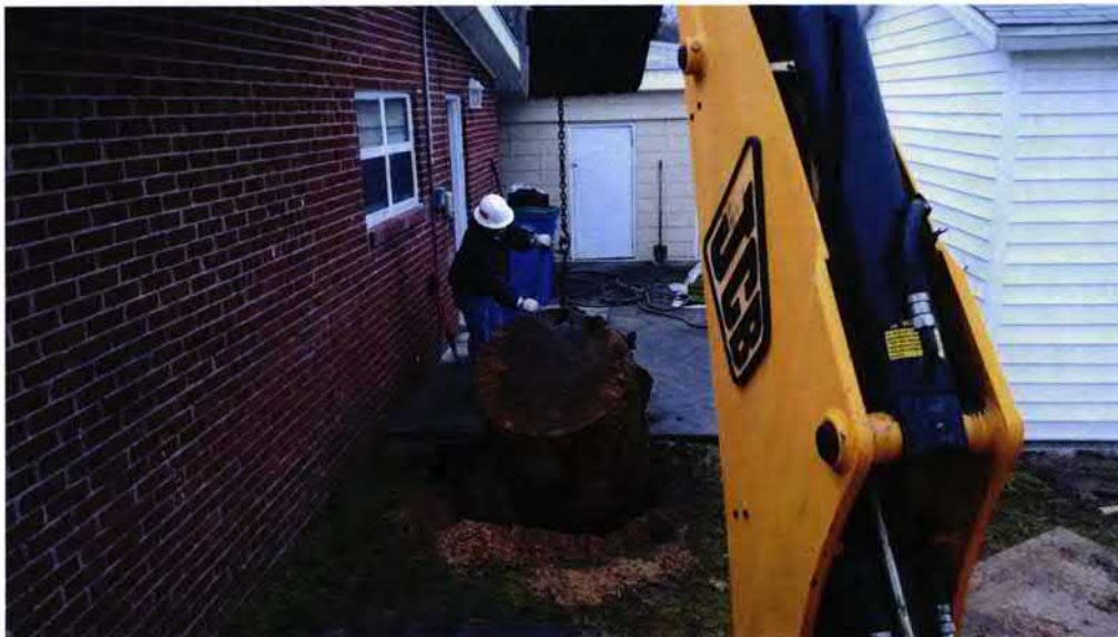
Picture 2: UST 689Camellia being lifted from the excavation.
